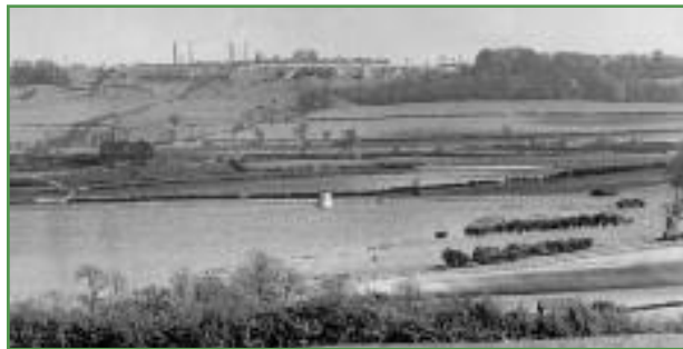
The recently constructed reservoir in the 1940s, with Corby steelworks in the background.
