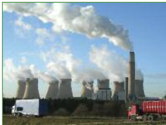
Freight lorries pass the coal powered Ratcliffe on Soar power station that provides electricity into the national grid. Local goods and micro-generation of renewable energy may play an increasingly important role in future.
