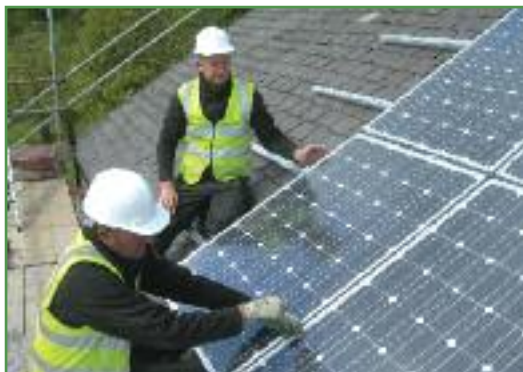
Photo-voltaic panels being installed on a local house.
